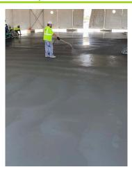
DuraForce(t) is a non-toxic, VOC free, topical liquid formulated to result in the creation of additional hydration products penetrating the multitude of capillaries, therefore densifying the slab during the curing process, providing an abrasion resistant slab and surface. Perfectly suited for:
